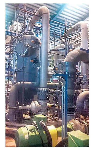
Condensate Polishing Plants (CPP) is designed for polishing of condensate of high pressure boilers and process heat exchangers in power plants and oil& gas industries. CPP treats physically the condensate that contaminated not chemically like once through Cooling Systems (On Shore Plants). Also CPP by utilizing coalescer filters, removes hydrocarbons contaminations in oil & gas condensates return from process heat exchangers.
