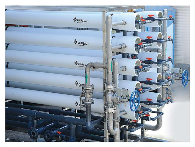
RO is a water purification technology that uses a partially permeable membrane to remove ions, molecules and larger particles from water. In reverse osmosis, an applied pressure is used to overcome osmotic pressure. Reverse osmosis can remove many types of dissolved and suspended chemical species as well as biological ones (principally bacteria) from water, and is used in both industrial processes and the production of potable water.
