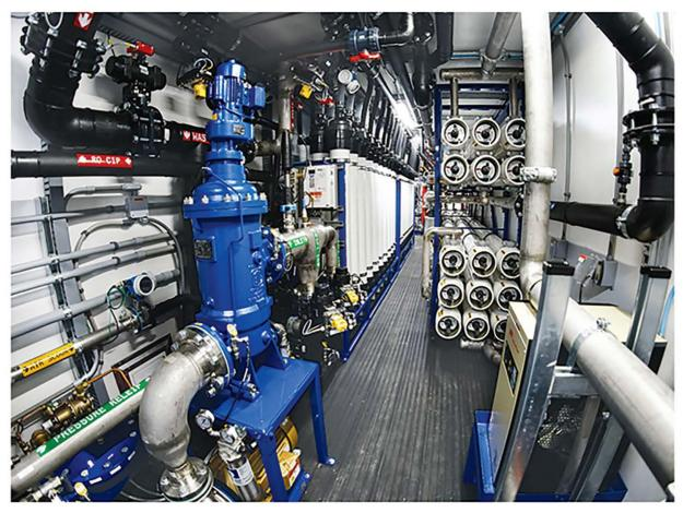
Mobile Reverse Osmosis (RO) & CEDI system produces demin water for temporary usage like pre-commissioning and commissioning period of plants. The system is assembled in truck container.
