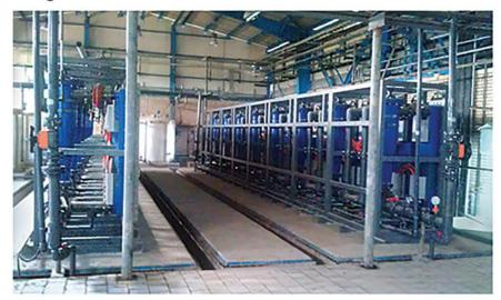
The Electro chlorination plant is designed to produce Sodium Hypochlorite (NaOCI) from seawater. Heavy duty, high performance cells use an injection moulded PVC casing and a bipolar electrode arrangement for maximum energy efficiency and Hypochlorite production. High quality coated titanium electrodes inside the electrolizer cell is utilized to achieve maximum cell operation life time. Indeed, reliable hydrogen removal system is designed to ensure safe operation of plant.
